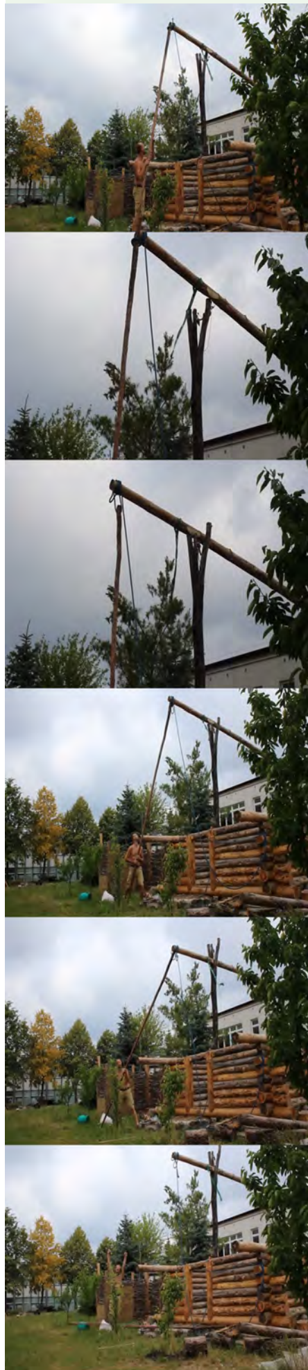
Fig. 9. An example of self-seating of a ridge in plow. A small mistake could ruin the whole day's work. As you can see during the work, the beam did not hit the socket. Fortunately, she stopped at the end of the opposite branch.
