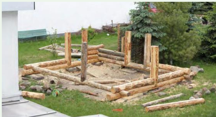
Fig. 3. The bottom logs placed on stone foundation with attached short logs.
