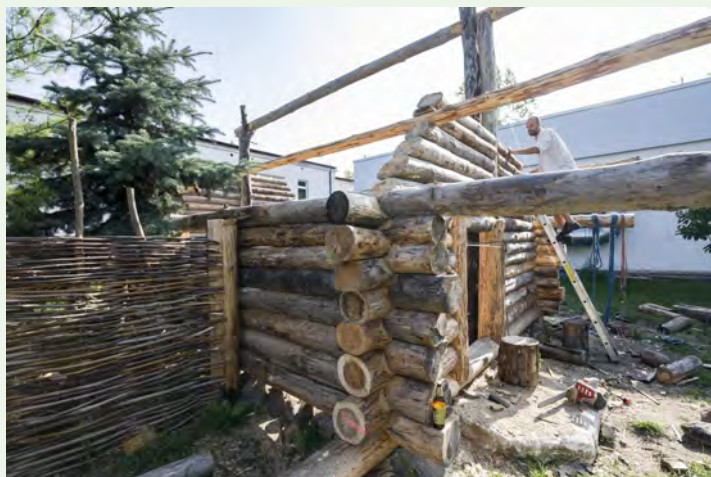
Fig. 6. Erection of the roof structure.
